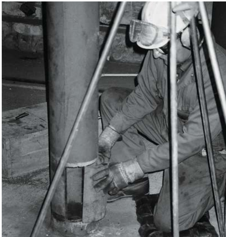
Above: Support column repair from beginning to end, using the Metalock process.
